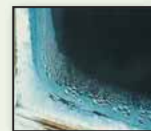
Window condensation fuels mold growth.
